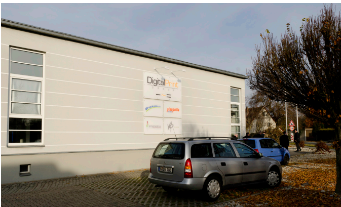
The Digital Print Group is housed in this building, not far from Nuremberg airport.
