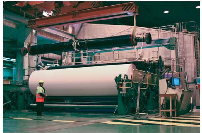
The main product from the M_Real Husum mill is copier paper, with over 240,000 tonnes produced here each year.
