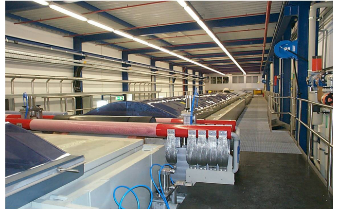
Another part of the manufacturing line (wet section) at Osterode.
