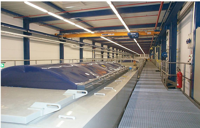
Part of the manufacturing line (wet section), at the Sonora plant in Osterode, Germany.
