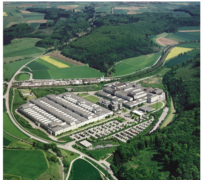
Heidelberg's Amstetten foundry sources more than 20% of its energy from renewable resources.
